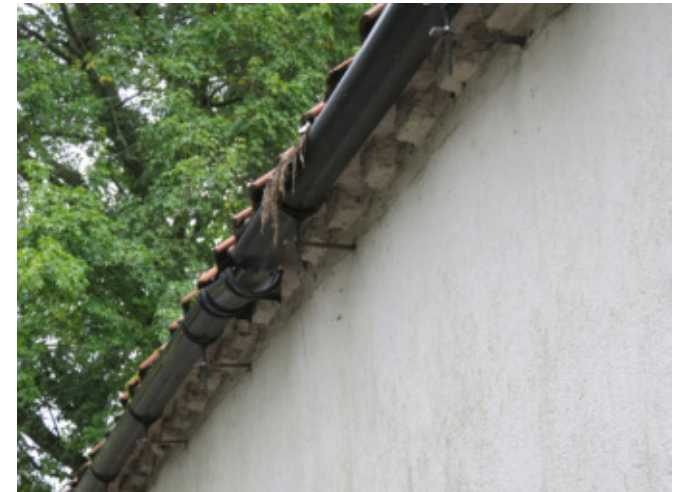
Broken gutters cause water to soak the walls, which leads to deterioration of the fabric
