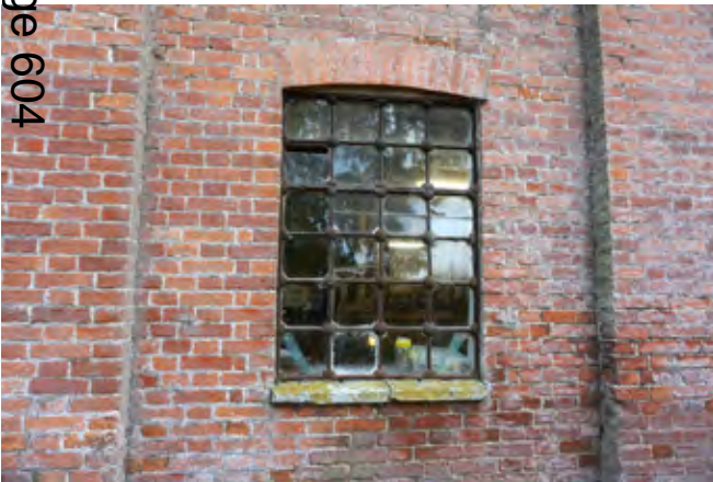
Rusted and bowed window on the mill
