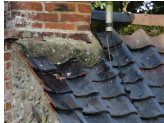
Inappropriate cementitious repairs to chimney and roof
