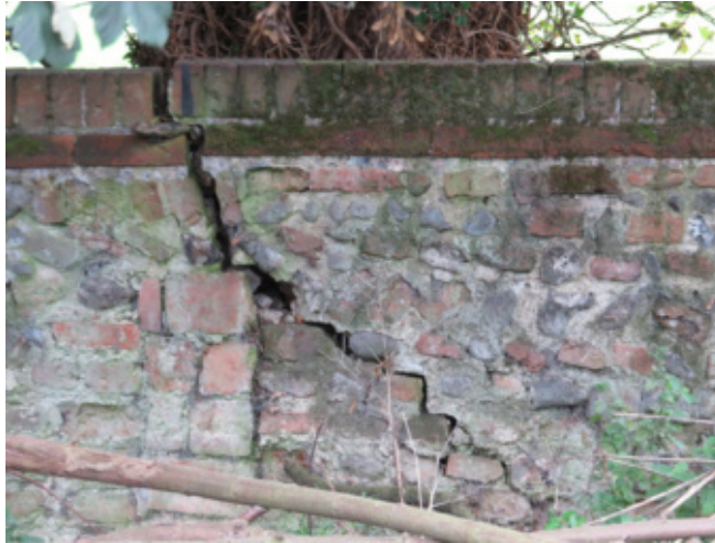
Cracked boundary wall due to tree growth
