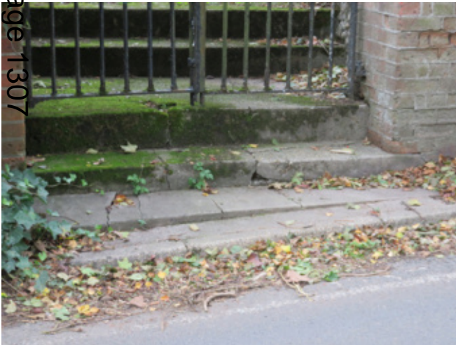
Cracking cementitious screed to steps
