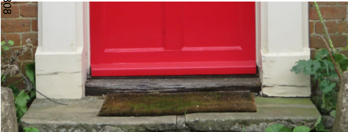
Rotting base to doorcase
