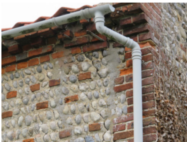
Cracks and cementitious repairs to a building
