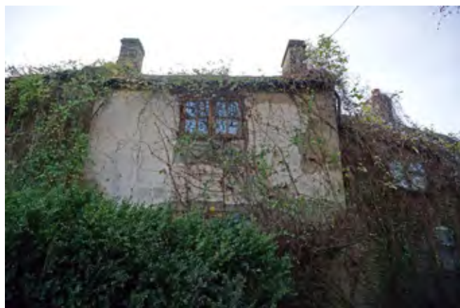
Cementitious render repairs
