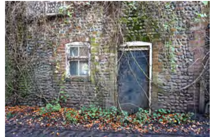
Timber work in poor condition
