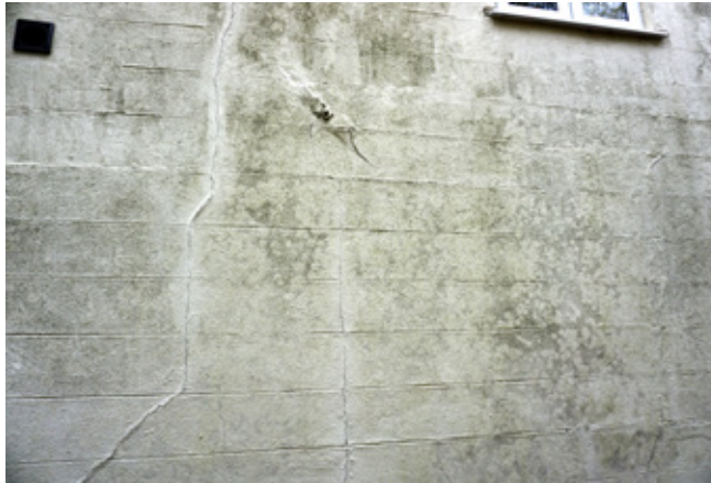
Cracked render and dirty paintwork
