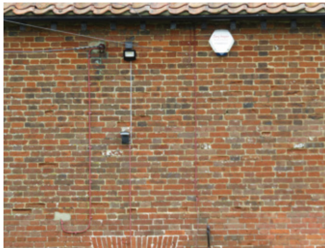
Accumulation of cables, light and security alarm
