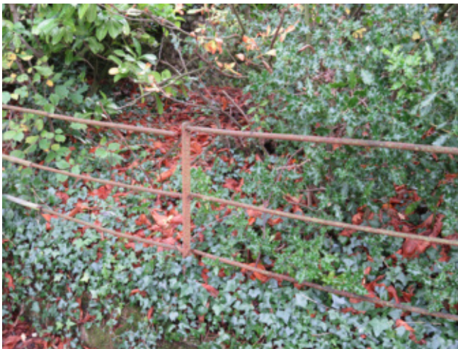
Broken and corroding railings
