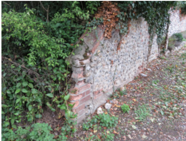
Damage to a wall compounded by cementitious pointing
