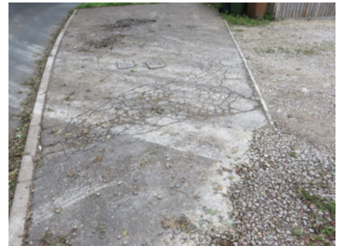
Poor surfacing to a large access splay
