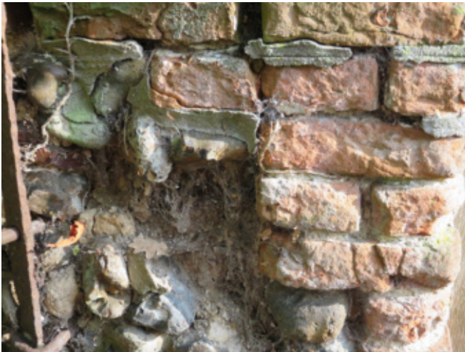
Excessive repointing, missing flints and damaged bricks to a historic boundary wall
