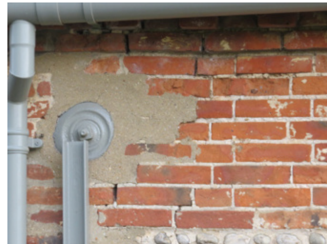
Cementitious repointing to brickwork
