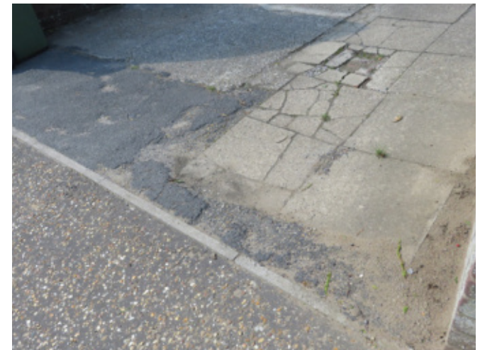
Cracked paving slabs on driveways
