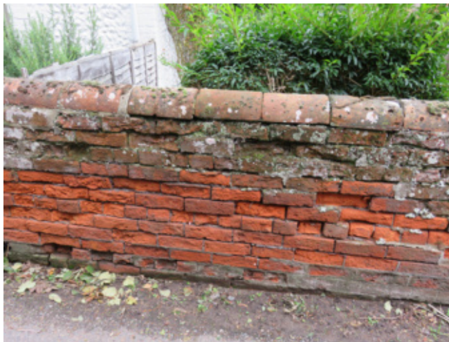
Boundary wall brick decay resulting from proximity to the road
