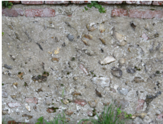
Excessive repointing to flint wall
