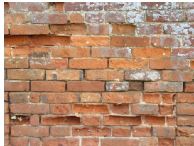
Eroding brickwork
