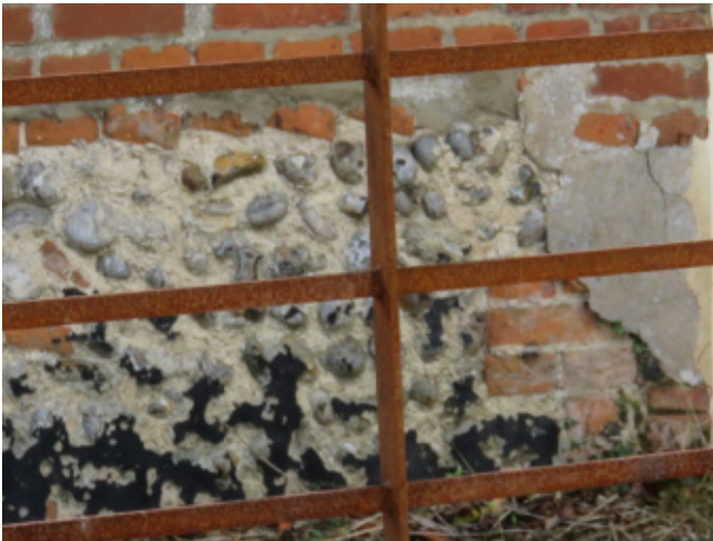
Inappropriate concrete repair
