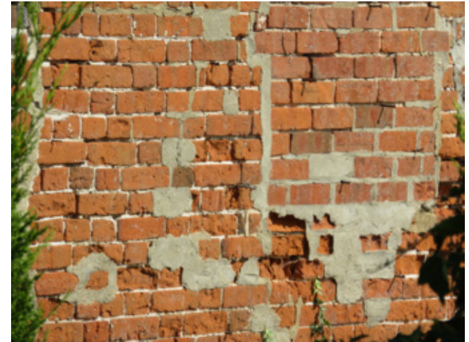
Eroded historic bricks due to cementitious pointing
