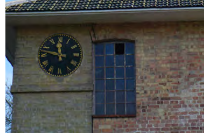
Rusted window frame with glass pane missing
