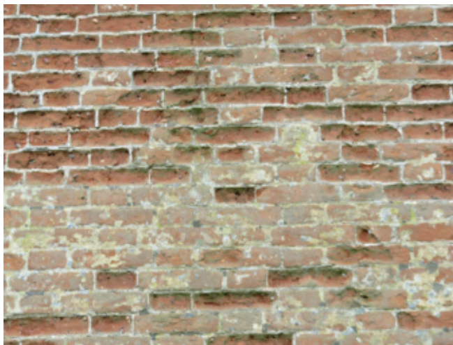
Brick delamination
