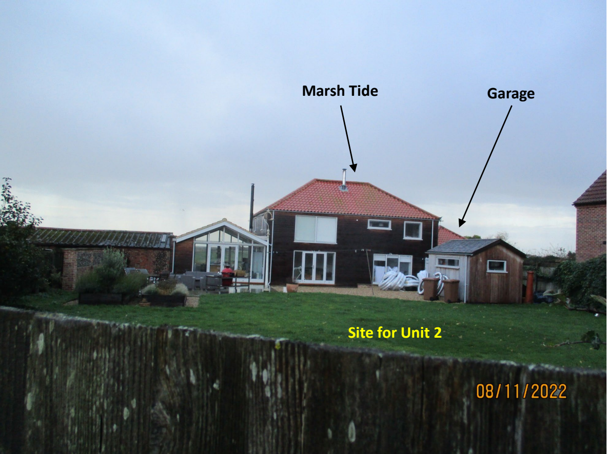
REAR (WEST) ELEVATION OF MARSH TIDE
