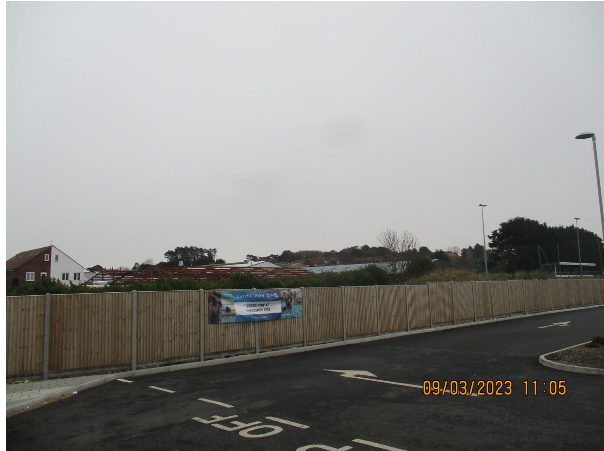
Looking to the South
