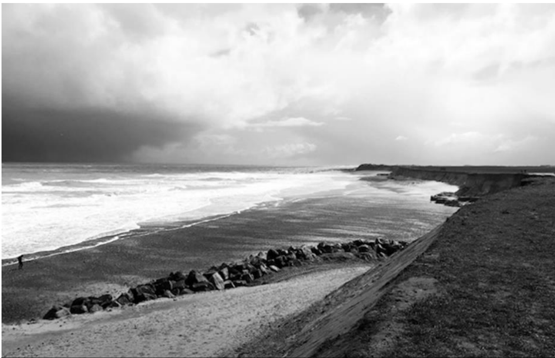
Risk Management Structure/rock berm at Happisburgh with cliff erosion shown.
