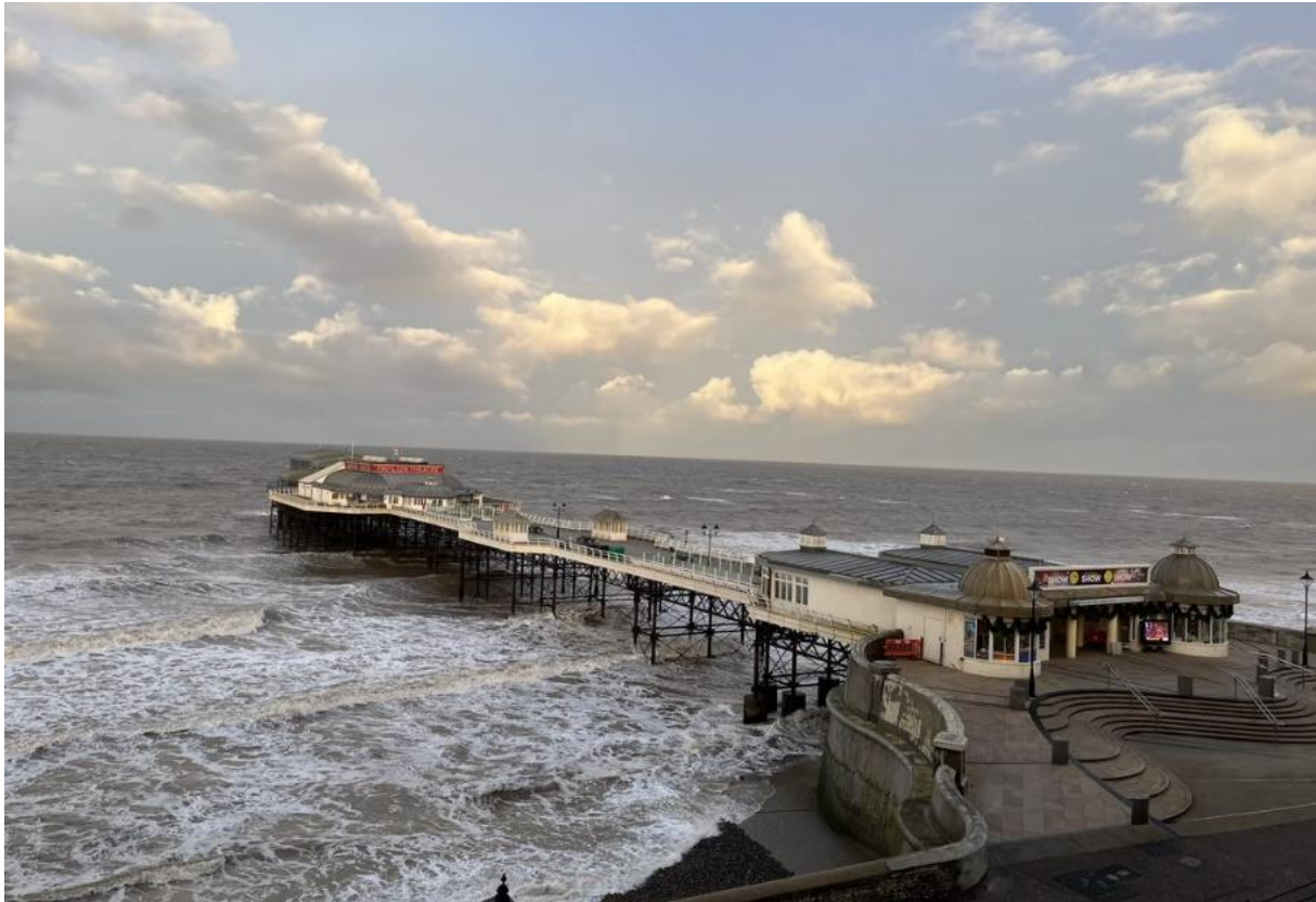
Cromer Pier with theatre, refreshments and lifeboat station in rough seas.
