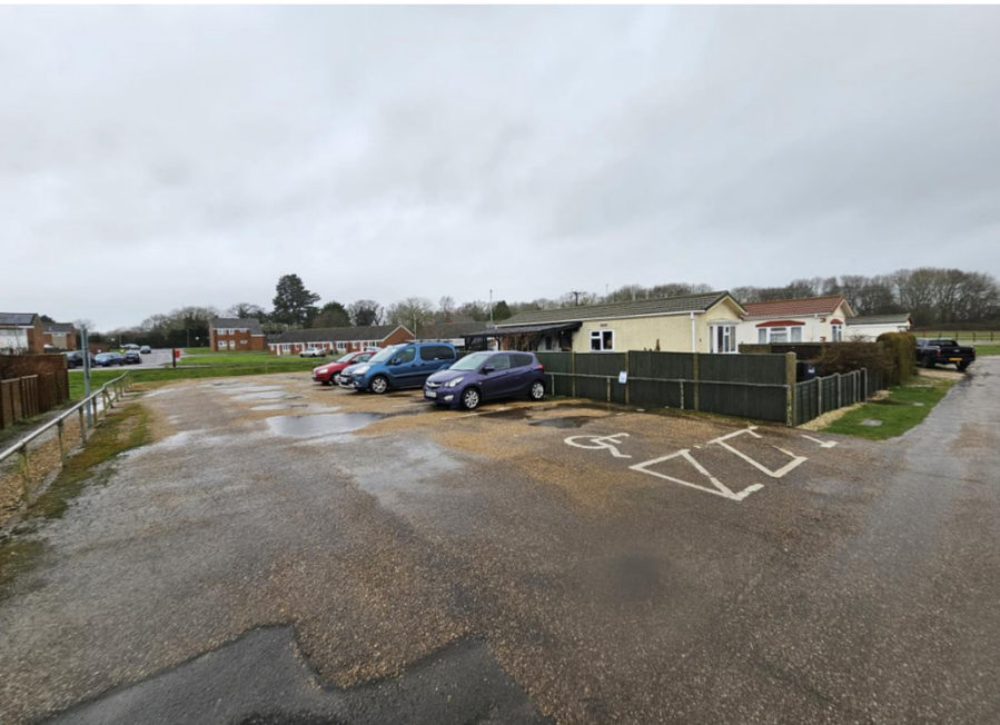
View westwards towards Green Lane Housing estate
