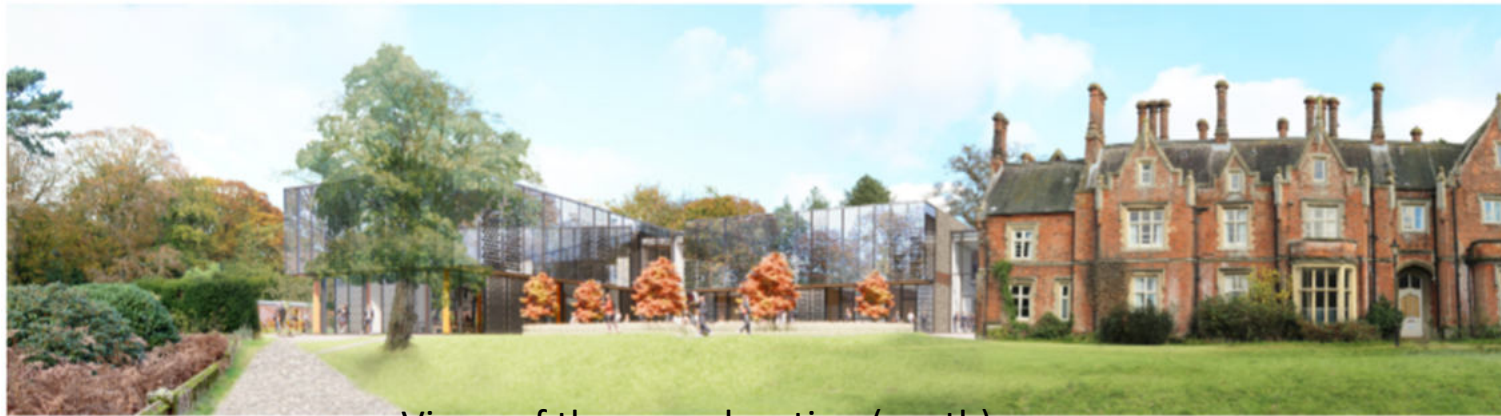
Views of the rear elevation (south)
