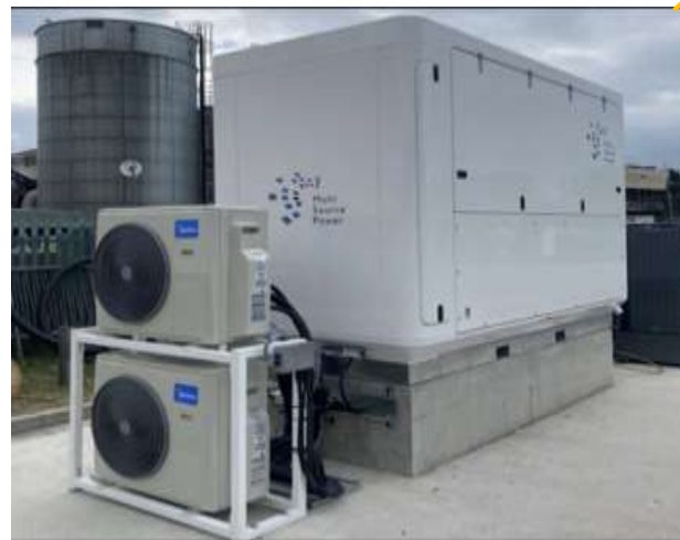
GRP units made up of the battery inverter and batteries
