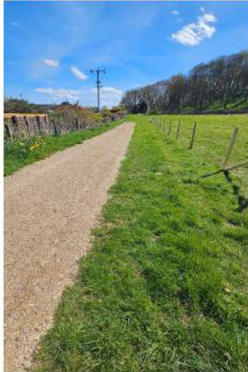
Finished Sub-Base S1
