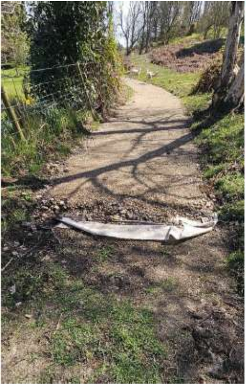
Geotextile & Sub-Base Make-up S1
