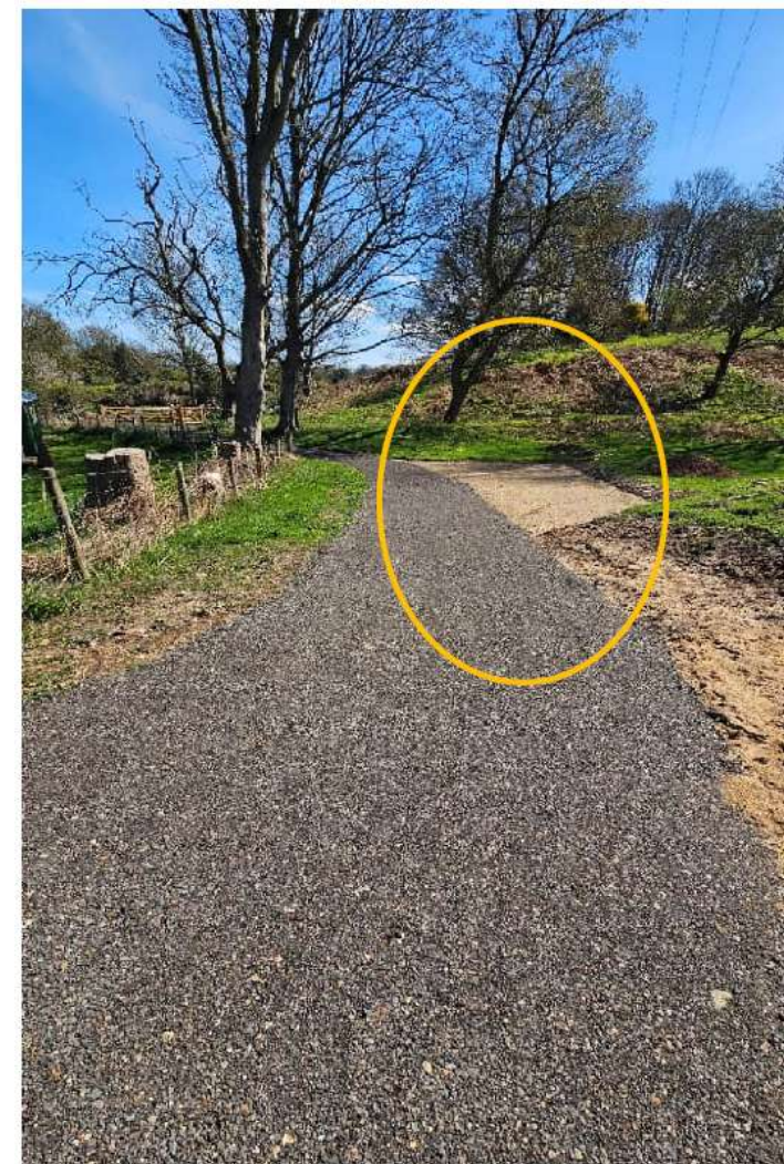
Sub-Base preparation for Rest Stop S1
