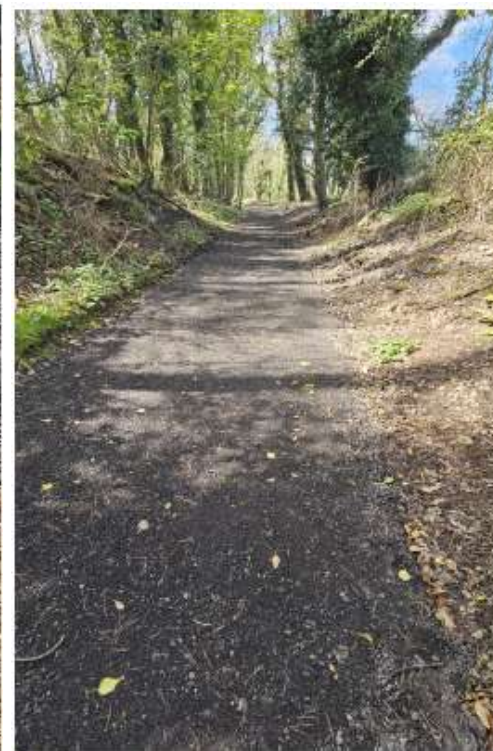
Finished Pathway S2
